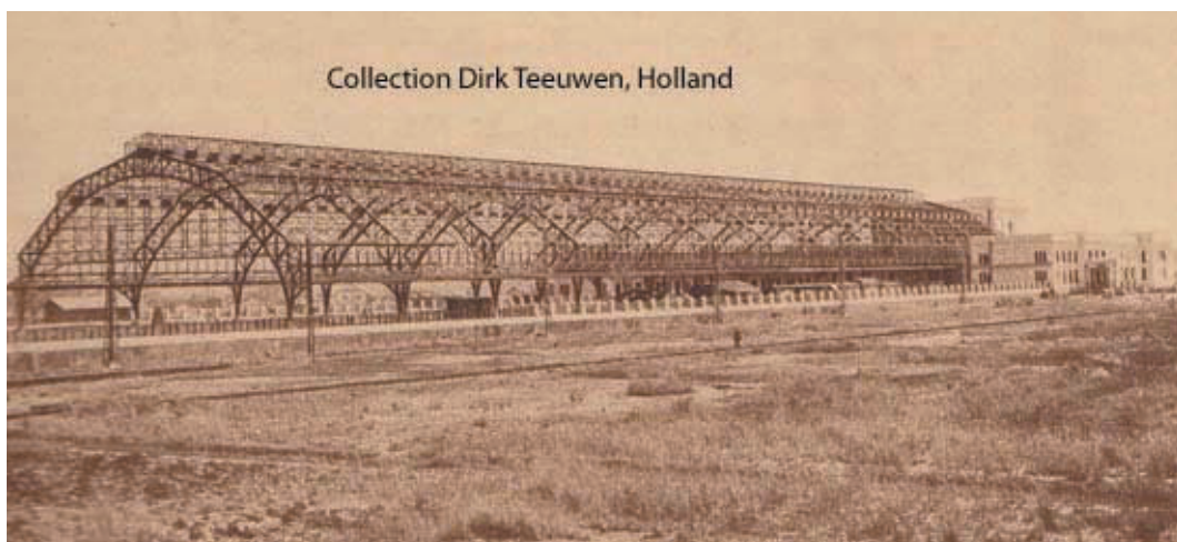
3.2 Roofing-in the new Tanjung Priok Railway Station; Batavia-Jakarta 1919
